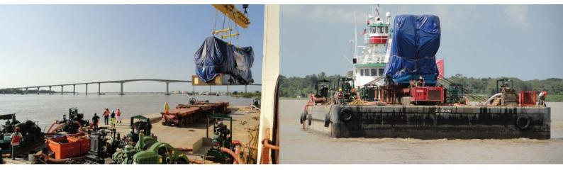
2 diesel engines of 300mT each ex Italy, 2 generators of 72mT each and 1 transformer of 52mT ex Finland had to be shipped, hauled and rigged onto foundations at the Staatsolie Power Company Surinam power plant on the Tout Lui Faut refinery just South of Paramaribo.
