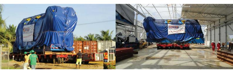
The engines were temporarily stored on the refinery roro dock and a few weeks later shifted on a 1,5 x Cometto SPMT onto their foundations.
