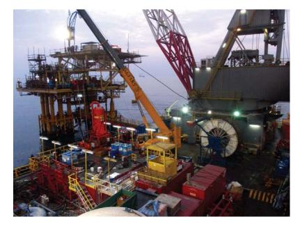
Several 8 point mooring plans were also provided to Aramco for approval. These mooring plans had to show the crane barge position at the platform, with emergency pull off methods, we also had to show in the mooring plan the location of buoys which were to be used to keep the mooring wires clear of all pipelines at the sea bed.
